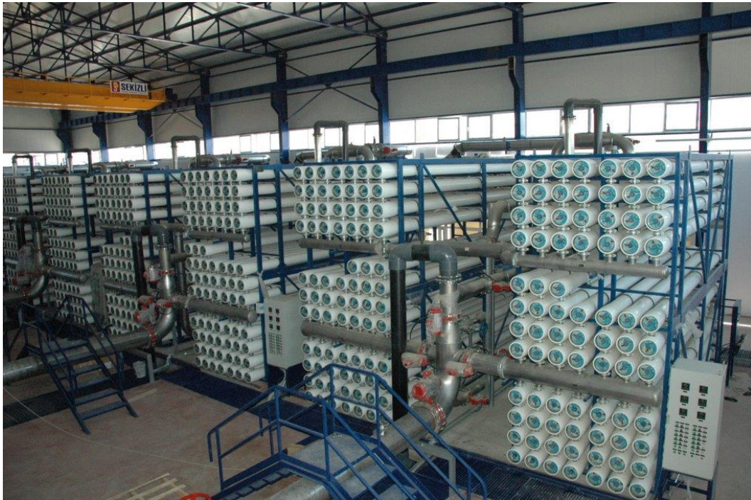
Figure 3.2. RO system of the present plant in Kirikkale city (Koyuncu et al., 2018)
