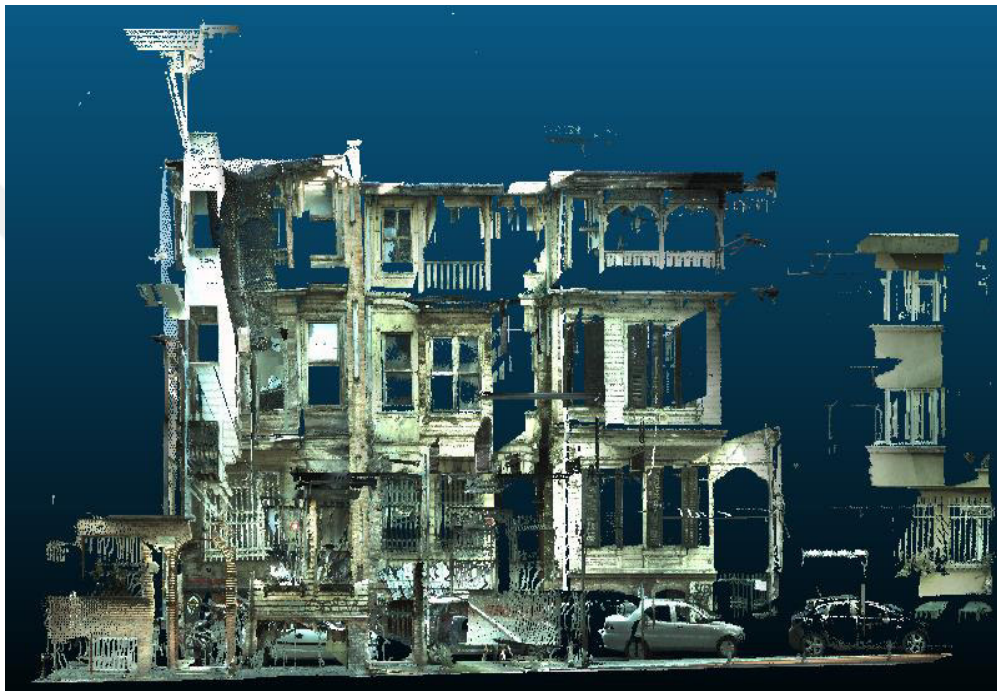
Figure 4.9. TLS Original view of a building front face
